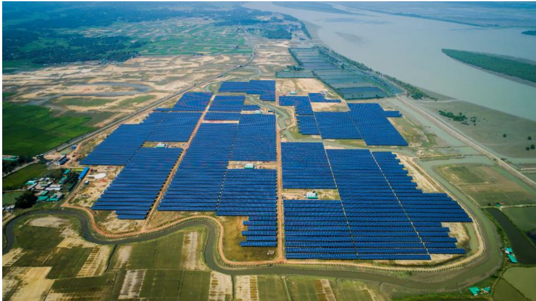
Photo 8: Aerial view of constructed TSEL
