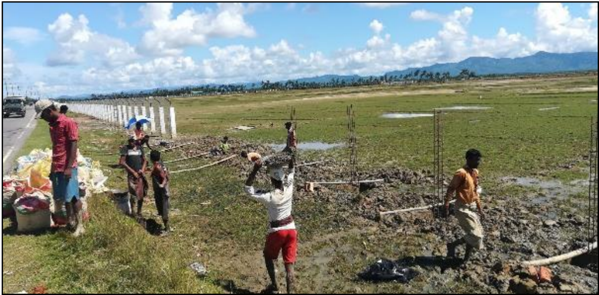
Photo 6: North Side of the Project Area
