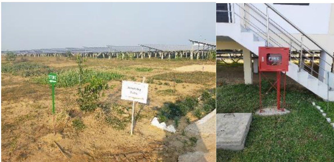
Photo 12: Designated Assembly Point for Fire Hazard and Fire Hydrant
